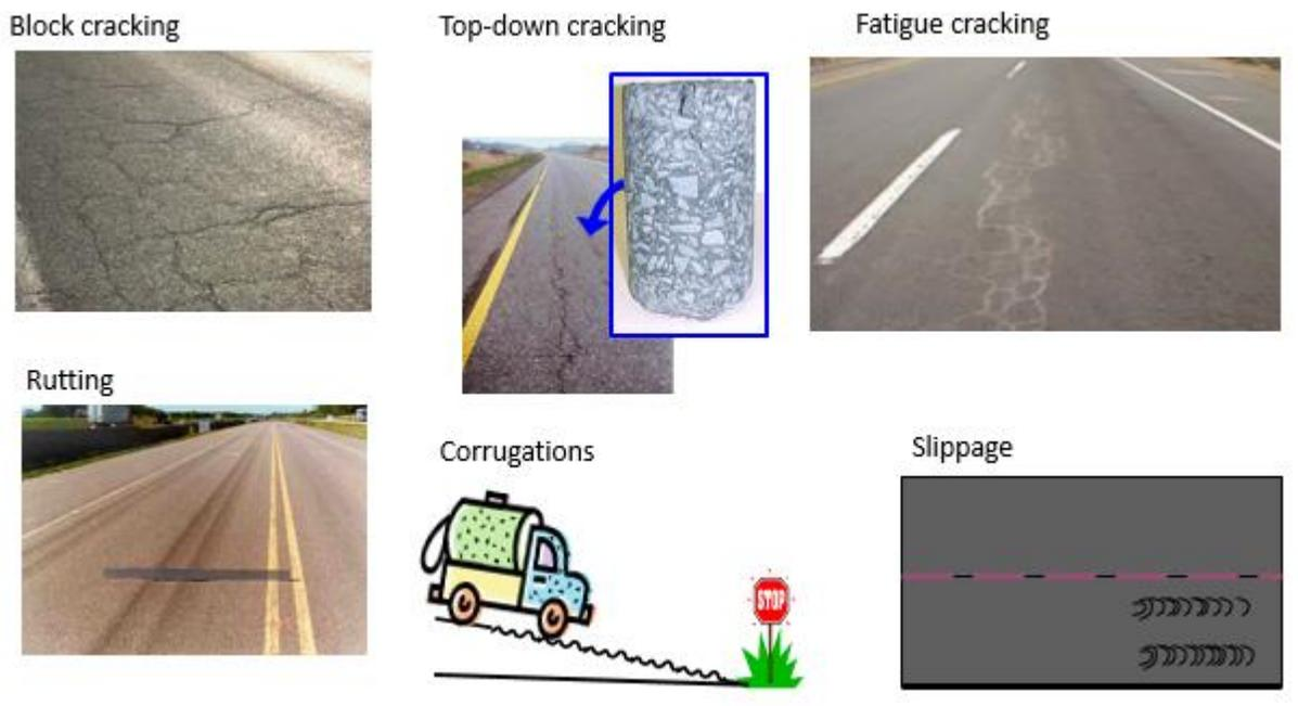
**Figure 3. Distresses in the HMA pavement.**
