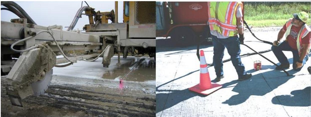
**Figure 10. Sawing and sealing joints.**
