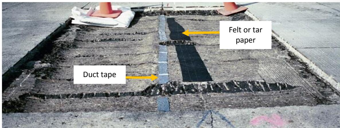
**Figure 6. Pre-overlay repairs and measures taken to reduce reflective cracking.**
