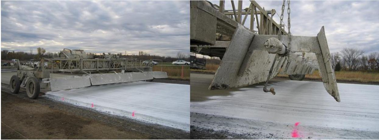
**Figure 9. Application of a curing compound.**
