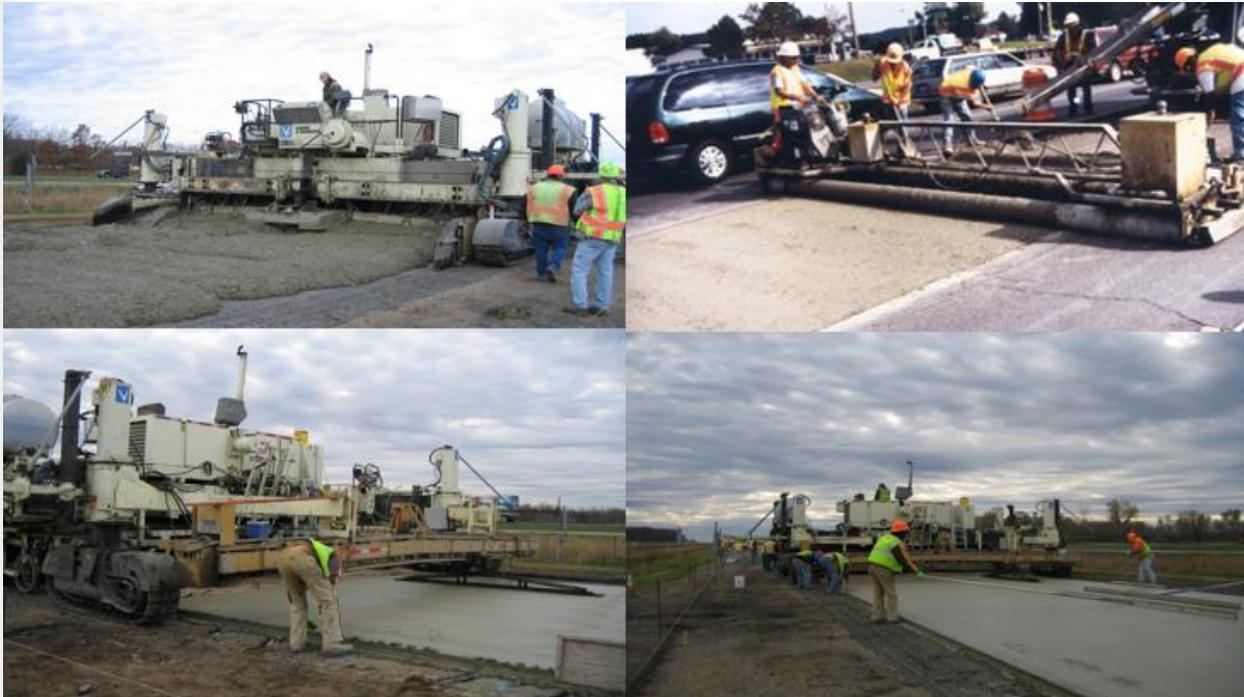
**Figure 8. Placing and finishing the BCOA.**
