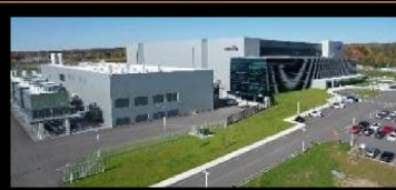
Marcy, NY Device Fabrication
