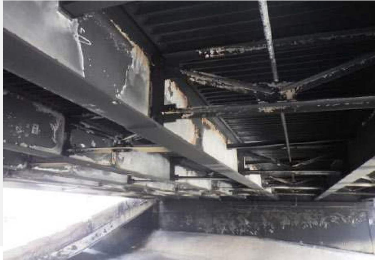
Underside of the southbound structure, looking back. Note the heavy soot staining
