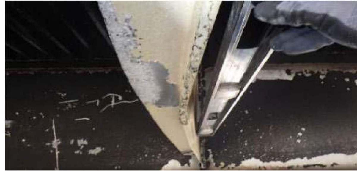
Severe cross frame distortion
