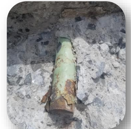
Corrosion damage
