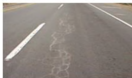
Fatigue cracking
