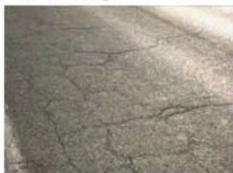
Block cracking
