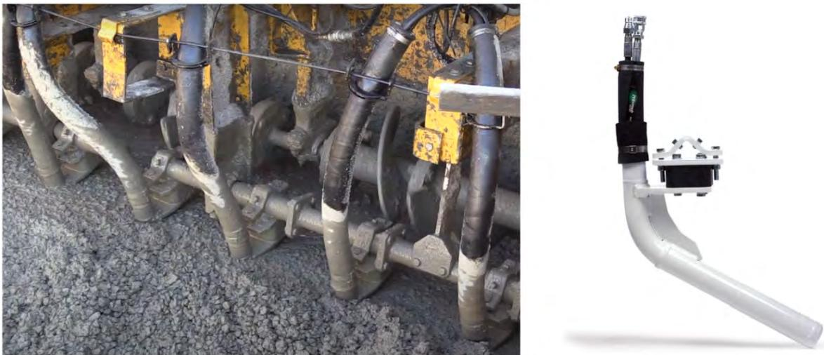
**Figure 1.** Slipform paving with typical concrete vibrator.
