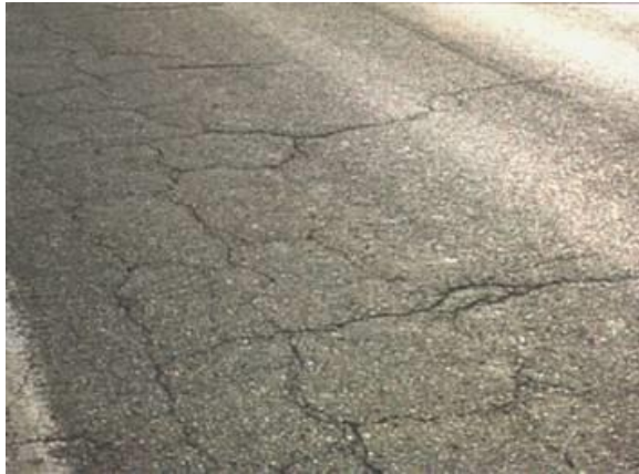
Top-down cracking
