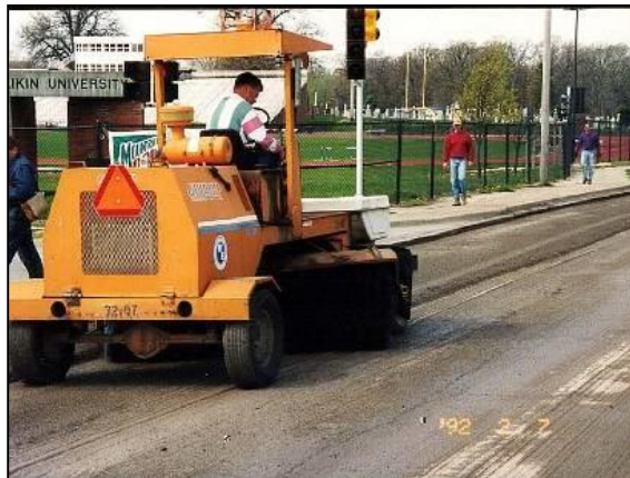
Figure 9. Sweeping the HMA surface after milling.
