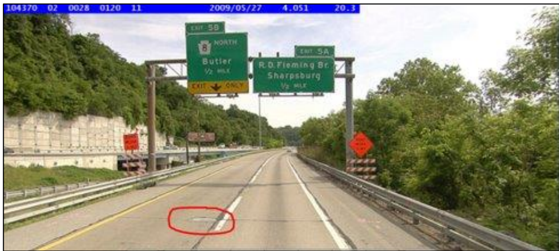
Figure 21: Condition in 2009, before MCR Corner Repair Source: Pennsylvania Department of Transportation
