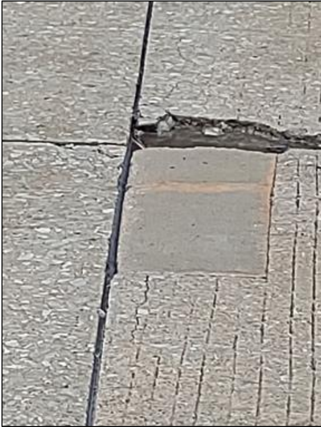
Figure 28: Route 22 Partial Depth Repair Intact
