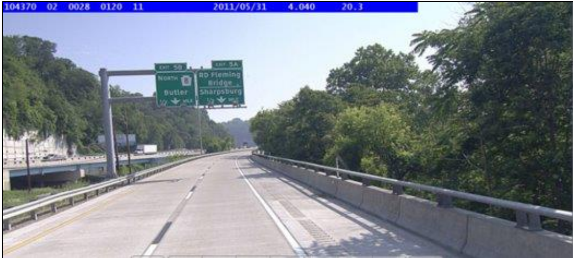
Figure 22: Condition in 2011 after MCR Corner Repair in 2010 and Reconstruction Source: Pennsylvania Department of Transportation
