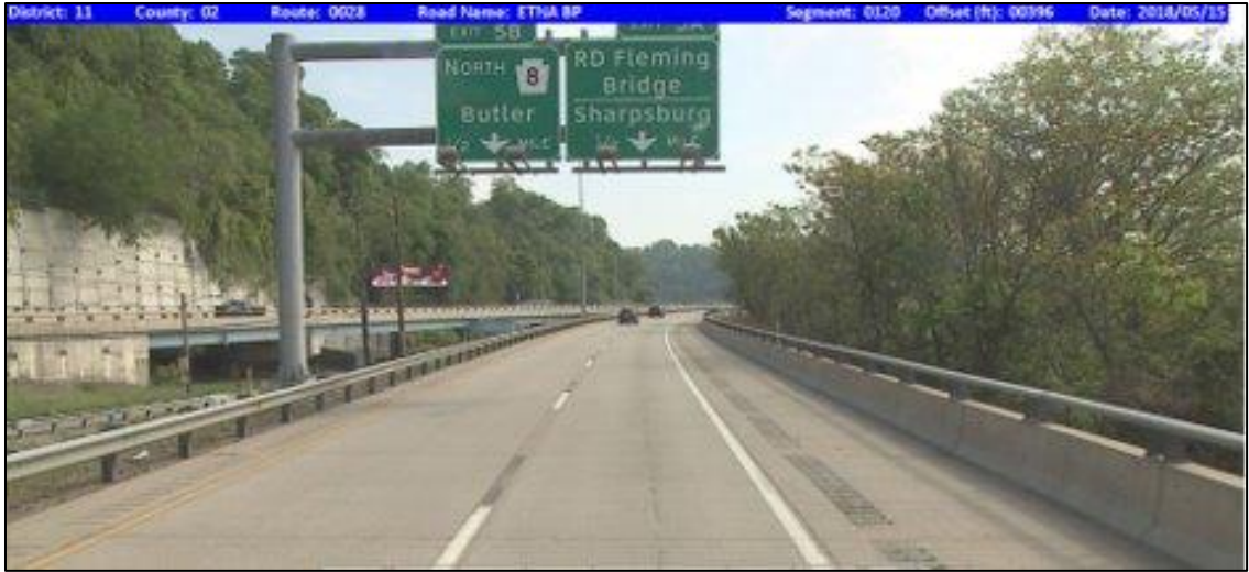
Figure 24: Condition in 2018 after Reconstruction
