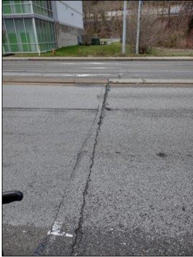
Figure 30: Route 51 Transverse Repair with Overlay Service Life of 3 Years
