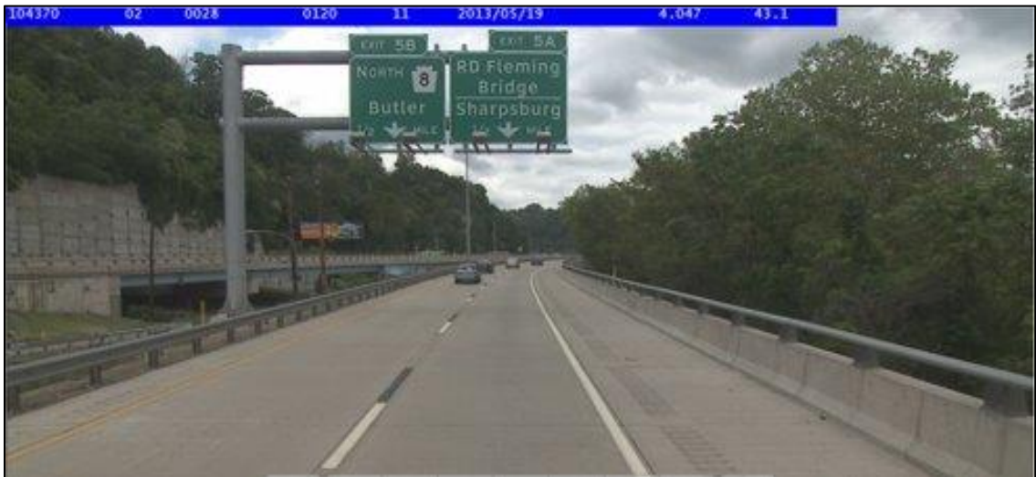
Figure 23: Condition in 2013 after Reconstruction Source: Pennsylvania Department of Transportation
