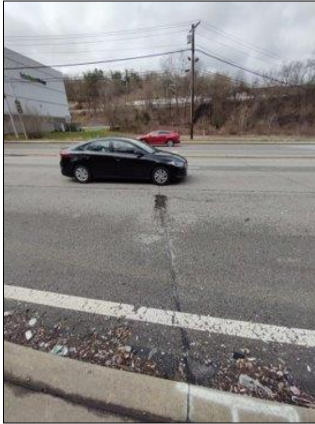
Figure 31: Route 51 Transverse Repair with Overlay Service Life of 3 Years
