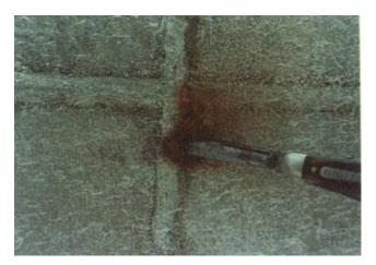
Figure 8. Weld Decay Corrosion [6]
