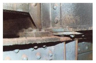
Figure 9. Fretting Corrosion at Stringer Joint [6]
