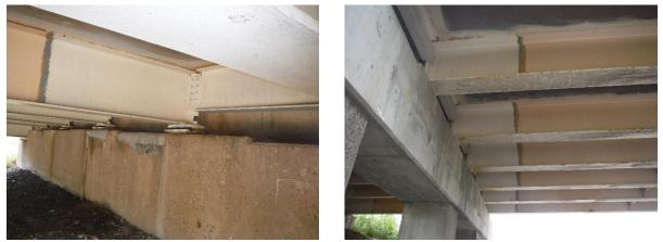
Figure 23 Polynox in girder ends of PA 136 Overpass over PA 51 after approximately 6 years of service
