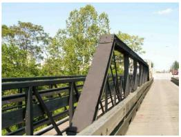
(a) Immediately after Painting (b) After 3 Years of Service Figure 29 Bollman Bridge in Williamsport MD immediately following application of Termarust and after three years of service [47]
