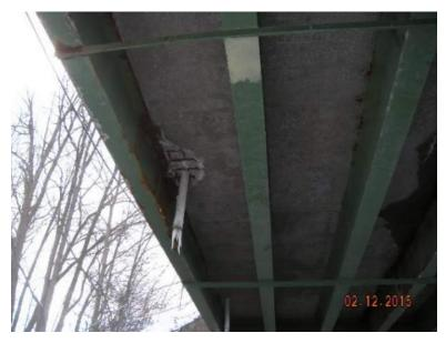
Figure 24 Improperly detailed free-falling scupper resulting in corrosion of bottom flange [41]
