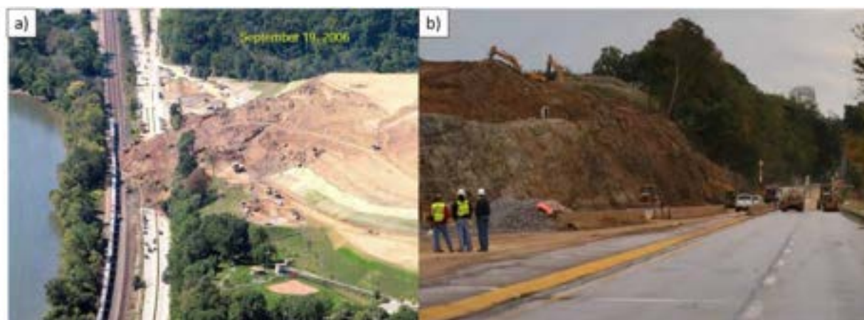
Figure 4.7.19. a) The September 19, 2006, Kilbuck landslide covered SR 65 and portions of the Norfolk-Southern main line railroad tracks is recognized as one of the region’s largest (Hamel, 2020); b) the remediation efforts took approximately 3 days to complete (Tribune photo).
