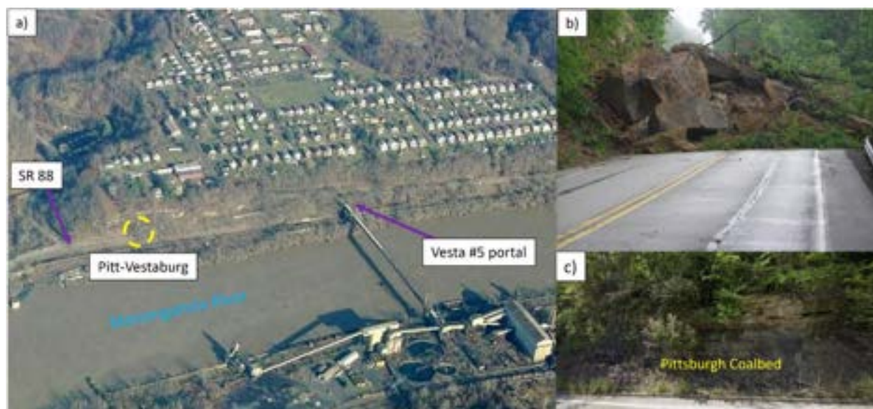
Figure 4.7.15. a) Location of the May 17, 2011, landslide along SR 88 (Photograph from Southwestern Pennsylvania Rural Exploration website); b) photograph of the massive Pitt-Vestaburg landslide (courtesy of Roy Painter); c) photograph of the Pittsburgh Coalbed alongside SR 88 near the Vesta #5 portal (Google Maps).
