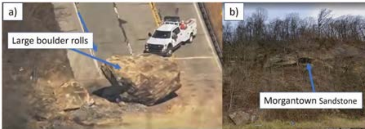
Figure 4.7.5. a) Location of the March 6, 2023, landslide (Photo from WTAE News); b) landslide material originated from an outcrop of Morgantown Sandstone above SR 837.
