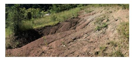
Erosion of Pittsburgh Redbeds along existing 3H:1V cut slope along I-79 near Neville Island
