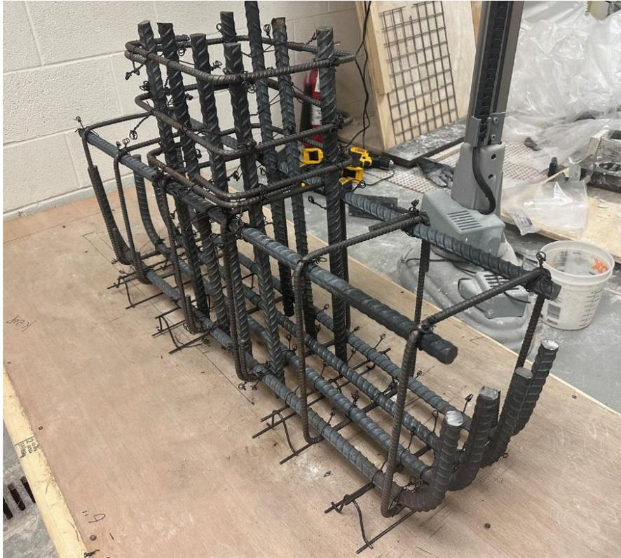
**Figure 13.** Reinforcing steel for pier cap
