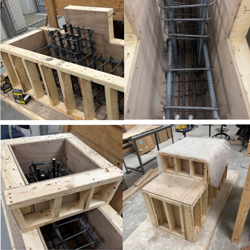
**Figure 14.** Conventionally cast prefabricated reinforced pier cap
