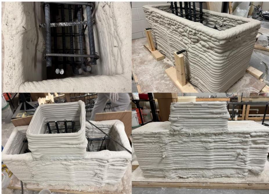
**Figure 16.** 3DCP of pier cap formwork
