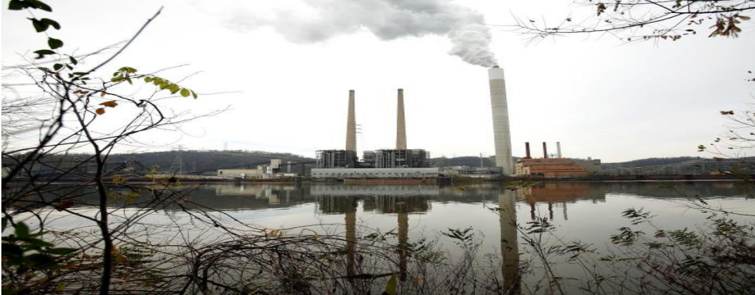
Mercury Removal from Flue Gas
